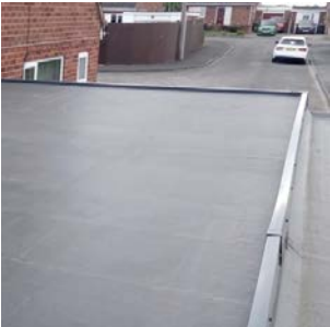
7. EPDM rubber roofing
